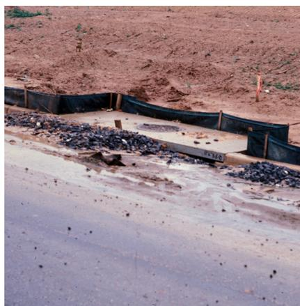
Sediment is the primary pollutant of concern associated with construction site stormwater runoff. Sediment-polluted stormwater can cause physical, chemical, and biological damage to waterways. Proper installation and maintenance of erosion and sediment control best management practices is essential to protect our waterways.
